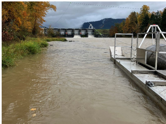
Figure H-19. Dexter Dam Tailrace at the old location (top) and the new location (bottom).
