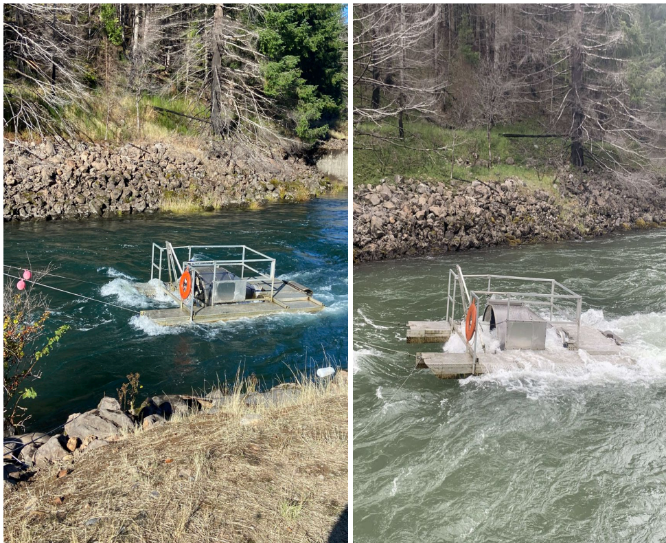
Figure H-9. Cougar Dam – Regulating Outlet at medium (left) and high (right) flow.
