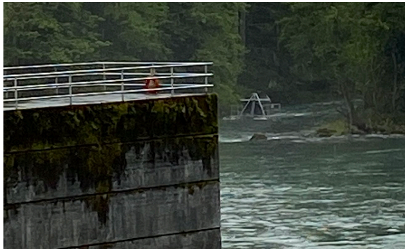
Figure H-17. Lookout Dam Tailrace – Spillway.
