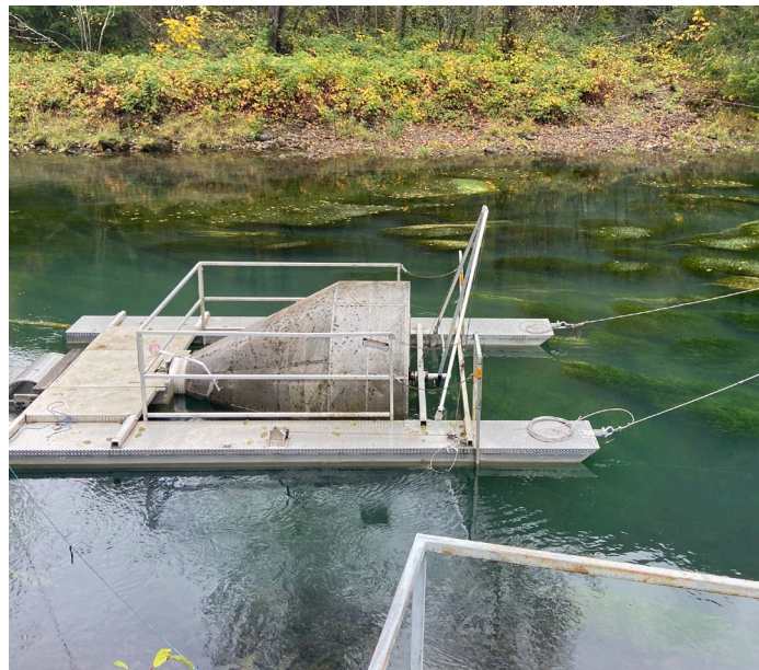
Figure H-15. Hills Creek Dam – Powerhouse Channel sampling at low flow.
